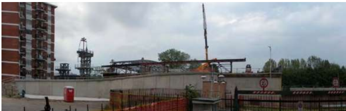
Fig.1. Covering of the A4 motorway
